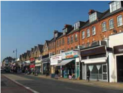
Red brick and yellow stock brick are traditional materials used in the area
